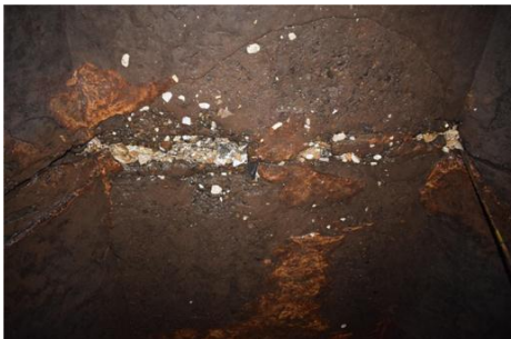
Figure 7: Rusting of Steel at Joint Location
