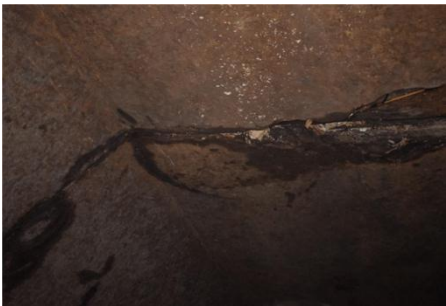
Figure 6: Leaking Joint with removed filling
