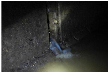
Figure 8: Opening of Joint with appreciable leakage between the Barrels 4 and 5
