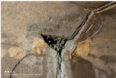
Figure 5: Damaged wall in Barrel No. 1 in Dry Condition (steel exposed)
