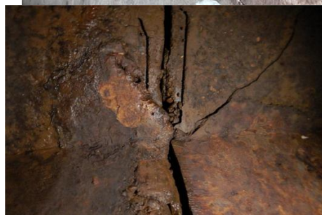
Figure 9: Deteriorated joint
